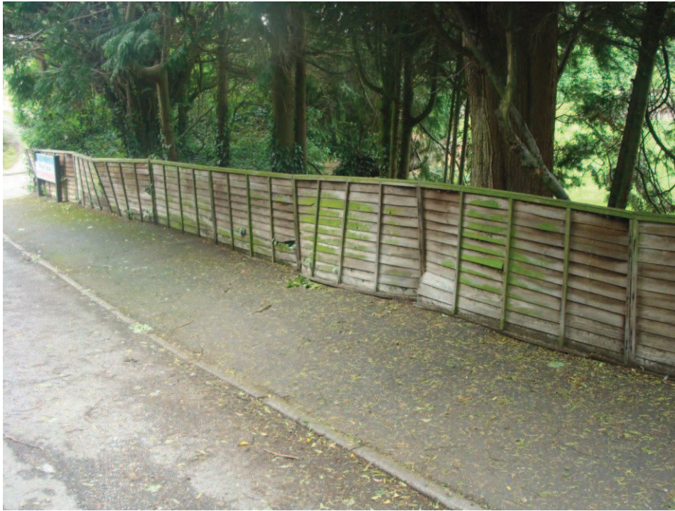
Picture 175. Deteriorating fence to front of Snowlands. This may need replacing in the future; an ideal solution would be with railings or hedge.
